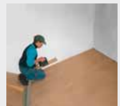
Hard board on top recommended
