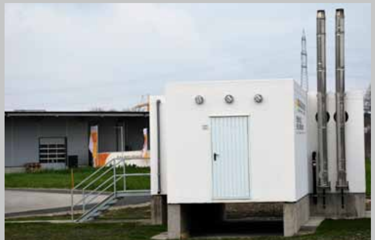
Two Single- Pellet Containers for a medium-sized business
